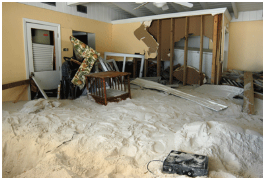
The storm surge of Hurricane Ivan (2004) pushed sand off of the shore of Pensacola Beach and into this Florida house. Image credit: FEMA/Mark Wolfe.
