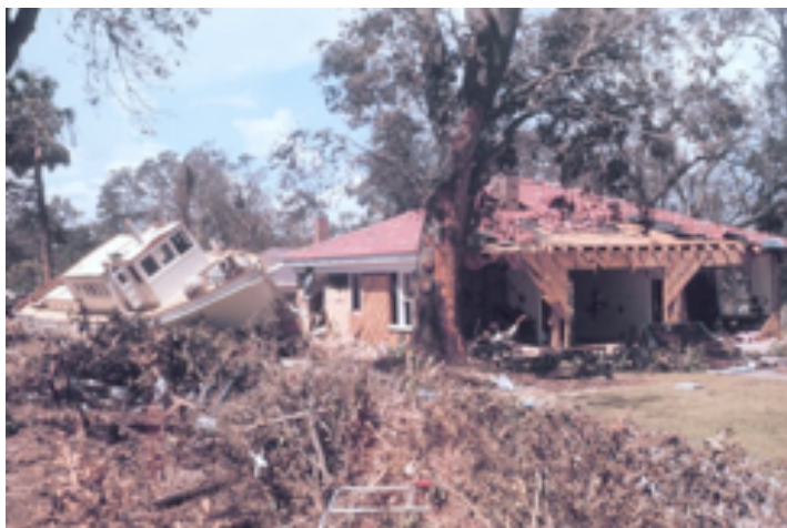
Damage from Hurricane Camille (1969) along the Mississippi Gulf Coast. Image credit: NOAA.
